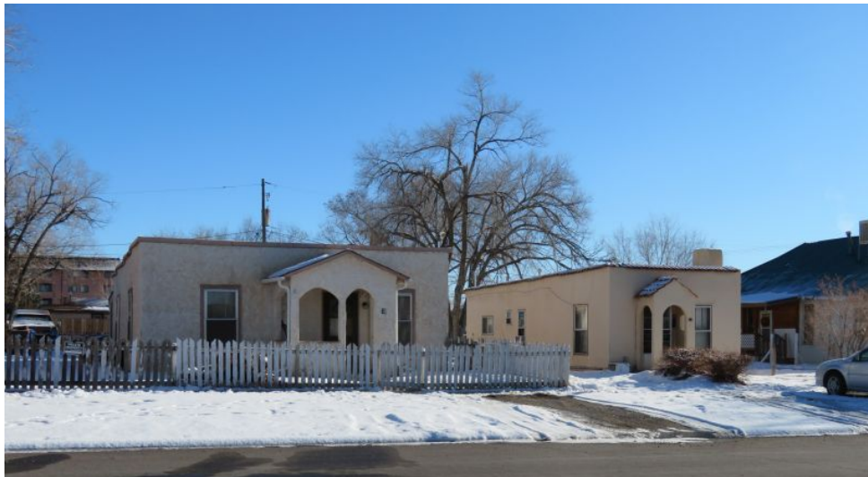
3031 Southeast Corner of North 4 th and Grand. Possible adobe construction with deep set one-over-one double-hung windows, turned porch posts, and hip roof with central chimney. Hipped-Roof Box style from the early 1900s.
