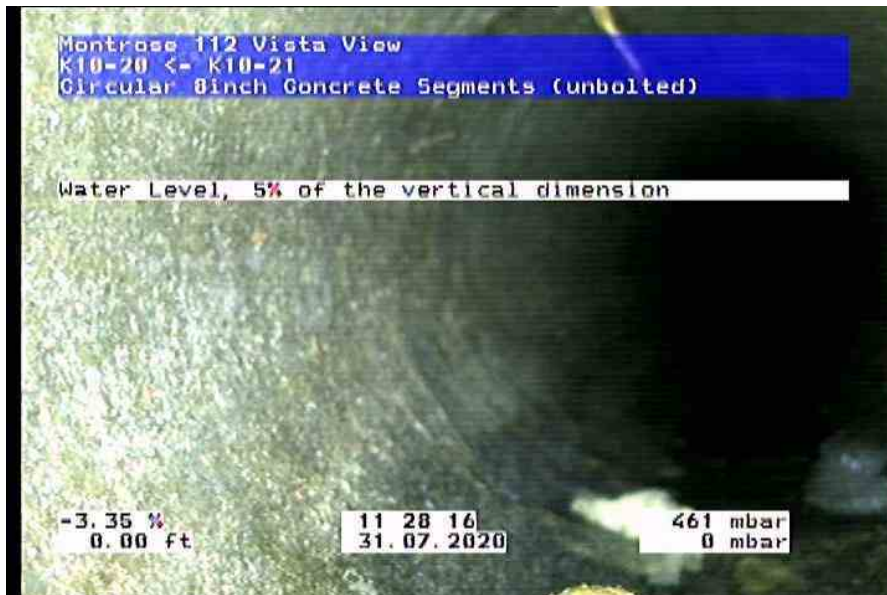
1896_474a487c-a1f2-489e-b782-a7f8d220e92a_20200731_113341_819.jpg, 00:00:23, 0.00ft Water Level, 5% of the vertical dimension
