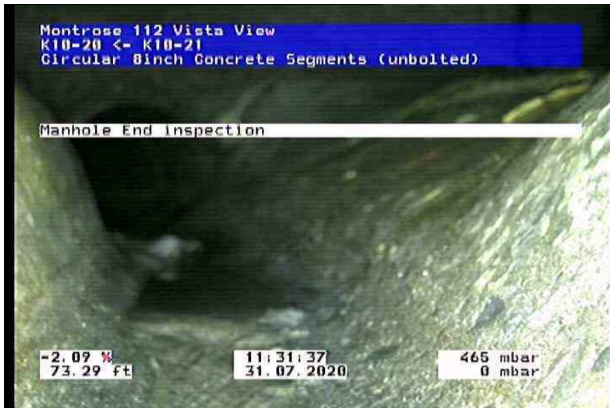
1896_ba736f81-90d9-48a1-860a-c0761a7de3ba_20200731_113703_035.jpg, 00:03:44, 73.29ft Manhole
