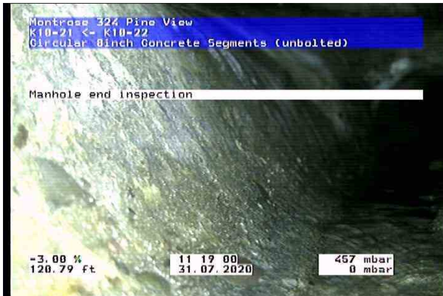
1755_0a125d37-9954-402b-b1fd-13467dfd608f_20200731_112425_278.jpg, 00:06:25, 120.79ft Manhole
