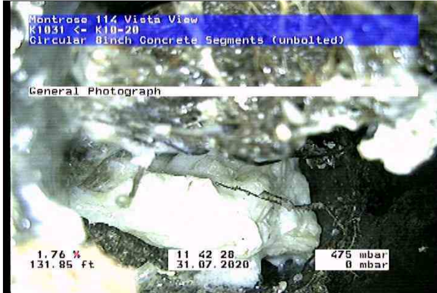
1740_4e800c32-e11a-482f-adf5-f5db7326430f_20200731_114753_574.jpg, 00:07:16, 131.85ft General Photograph
