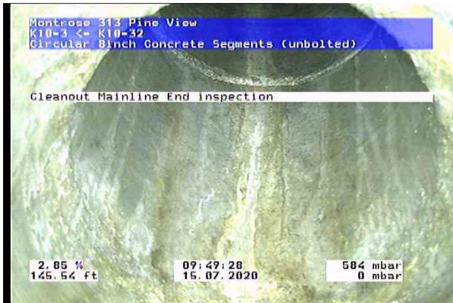
1843_930ce9b3-5e1d-4c46-aa2e-9cb4eb2c4d7c_20200715_095452_941.jpg, 00:15:12, 145.54ft Cleanout Mainline
