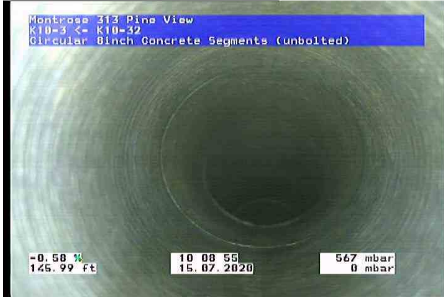
1843_88fb5202-8fa4-4720-a7c7-24b0b14790df_20200715_101419_747.jpg, 00:15:12, 145.54ft Cleanout/Mainline
